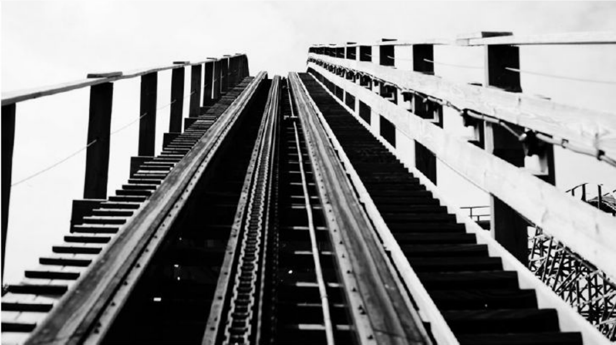
That undeniable "clack-clack-clack" sound you hear as a roller coaster train ascends the first lift hill comes from the chain that pulls up the cars. DAN CONSTIEN / EYEEM
